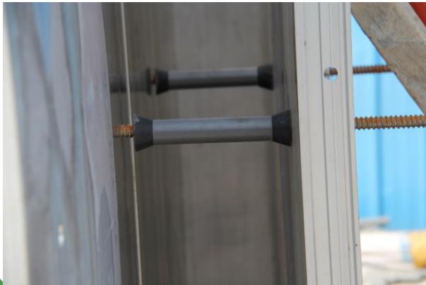
Screw tie rod system
