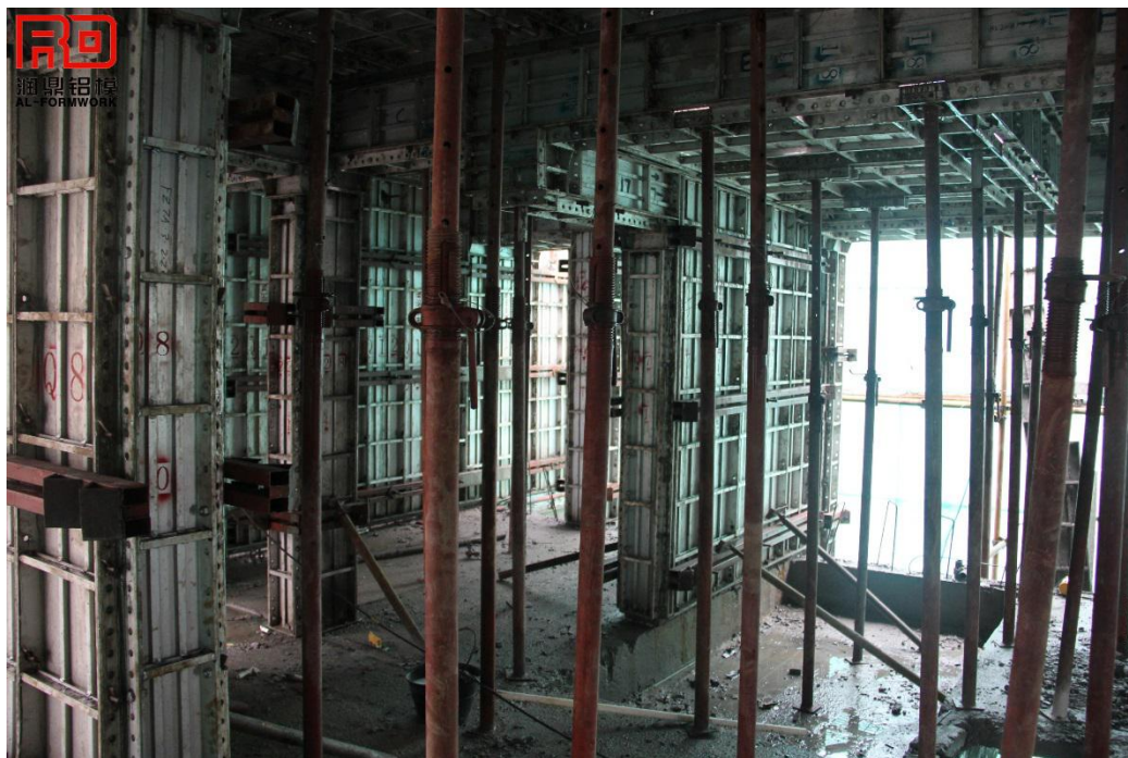
Supports for aluminum formwork system
