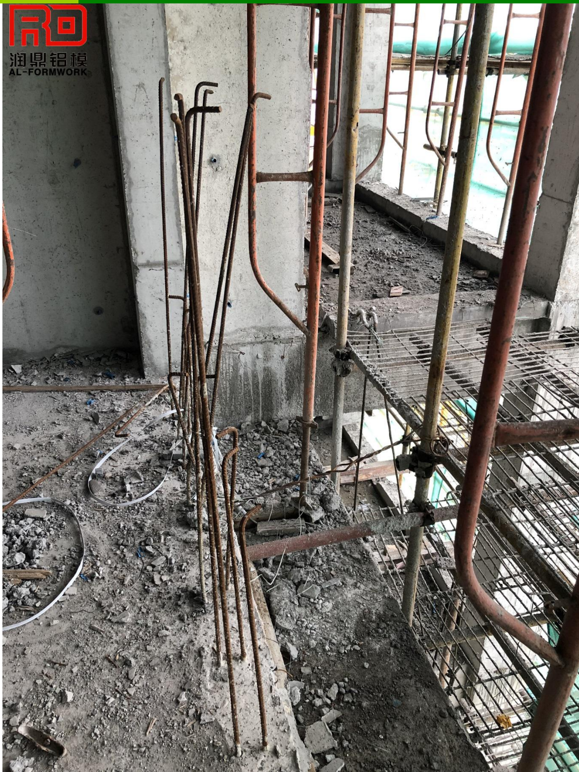
Steel bars reservation are waiting to be bound and made second concrete pouring, in plywood project.
