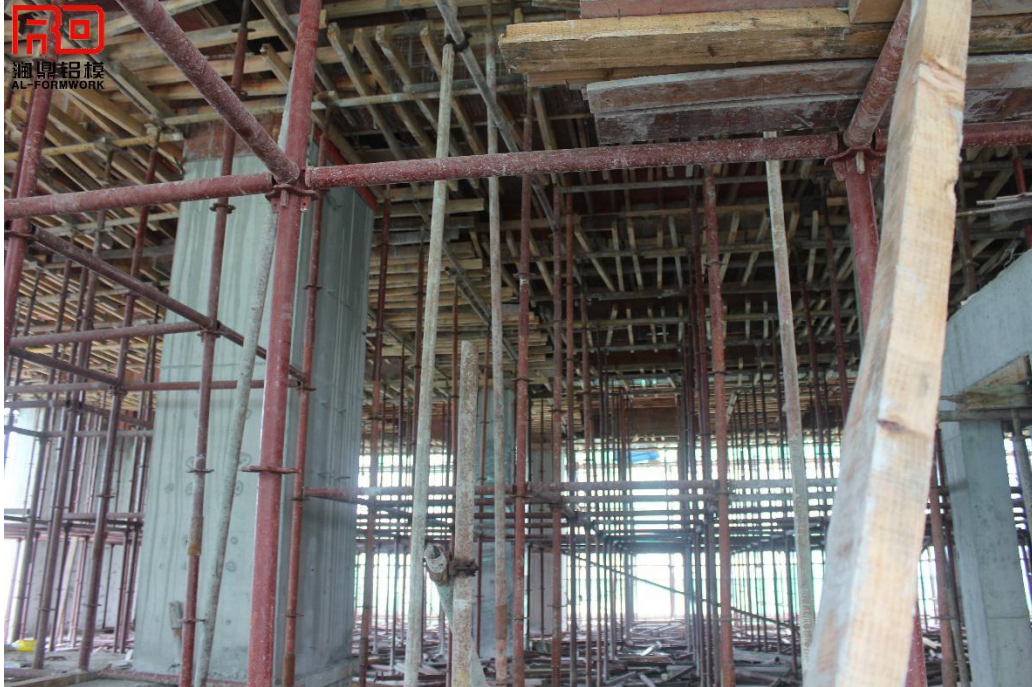
Supports for plywood formwork system
