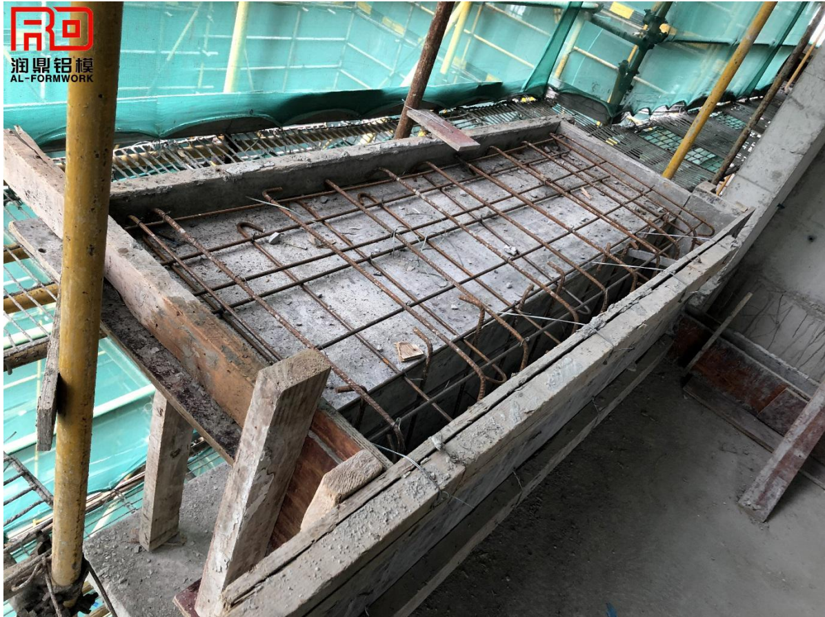
Waiting for the second concrete pouring
