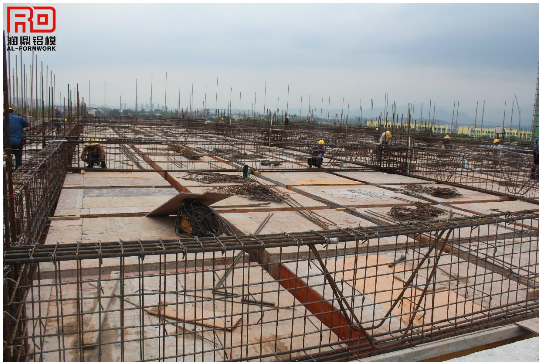
Binding the steel bars on the slab in plywood project
