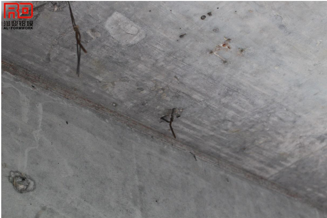
Iron nails stayed on the concrete surface.
