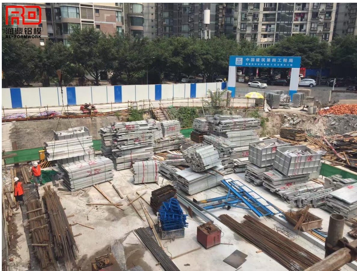
Aluminum formwork in storage of work site.
