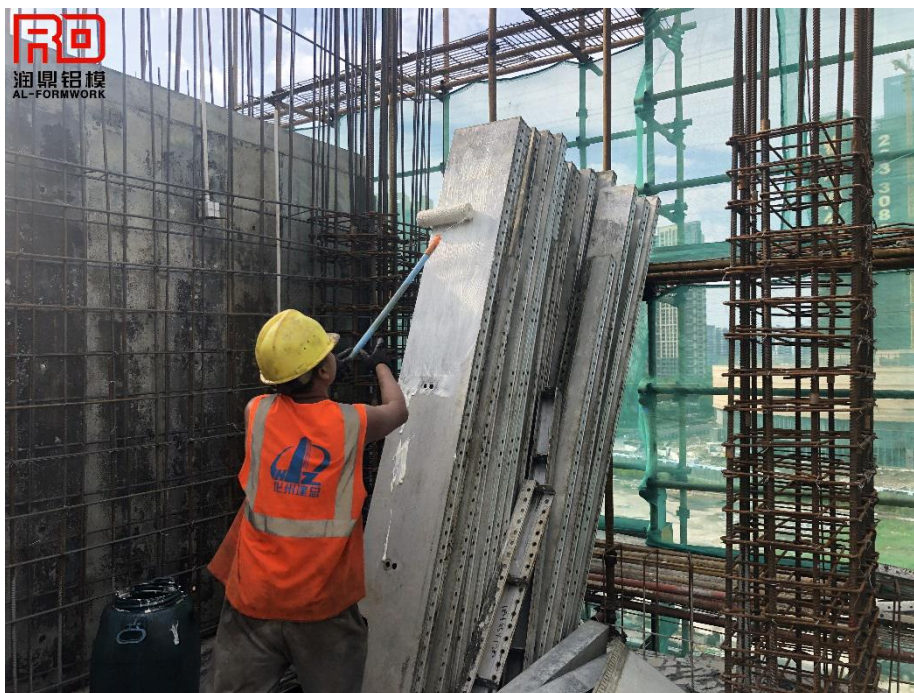
Coating the demoulding agent.
