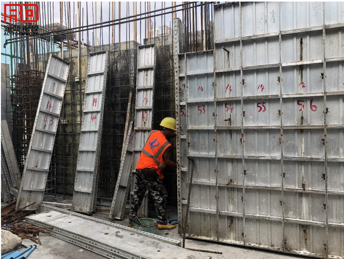
Steel wedge pins are locked on each aluminum panels.
