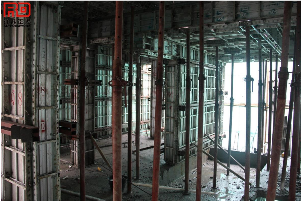
Supports for aluminum formwork system
