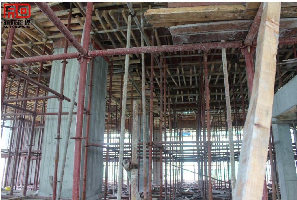
Supports for plywood formwork system
