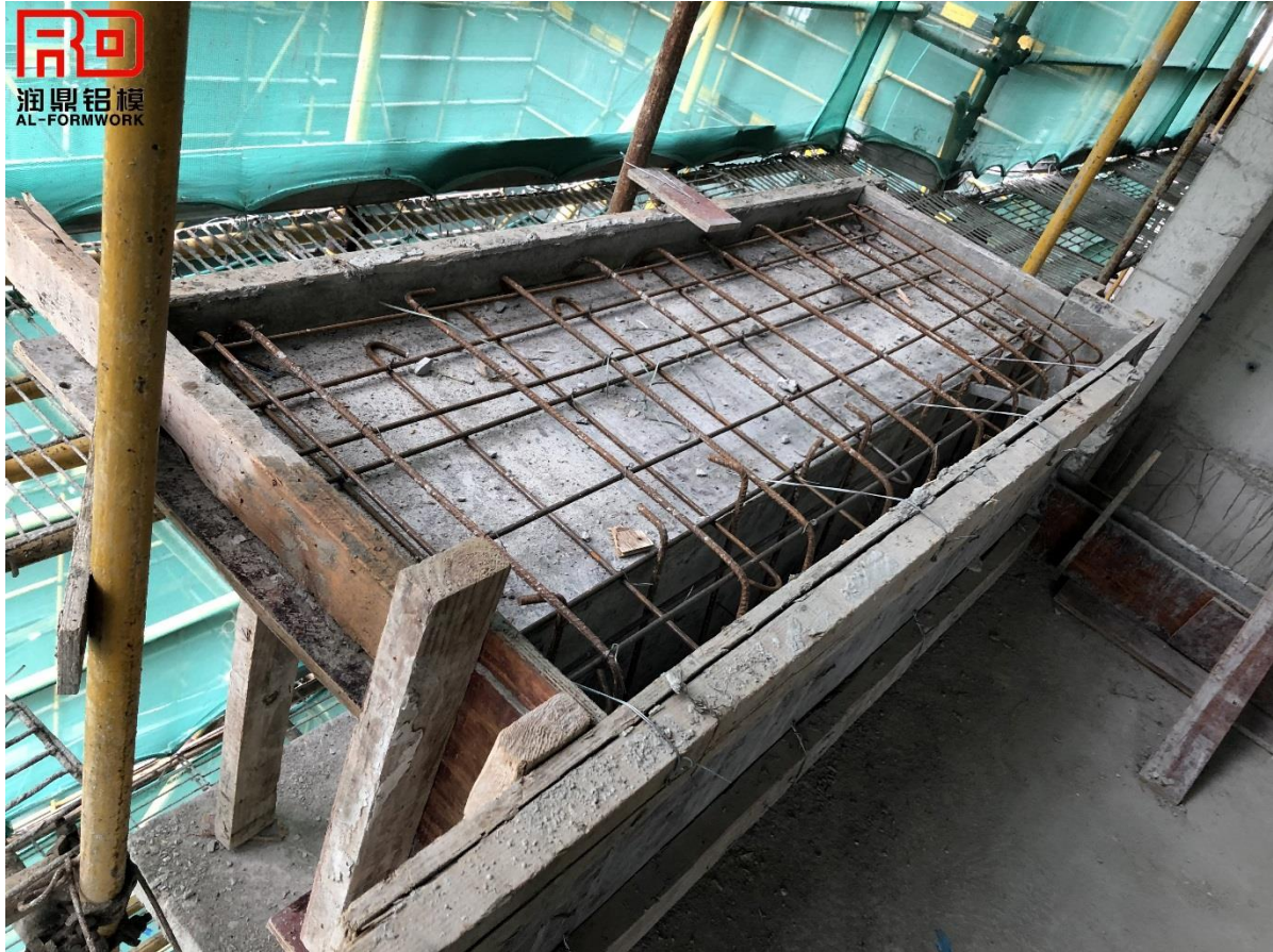
Waiting for the second concrete pouring
