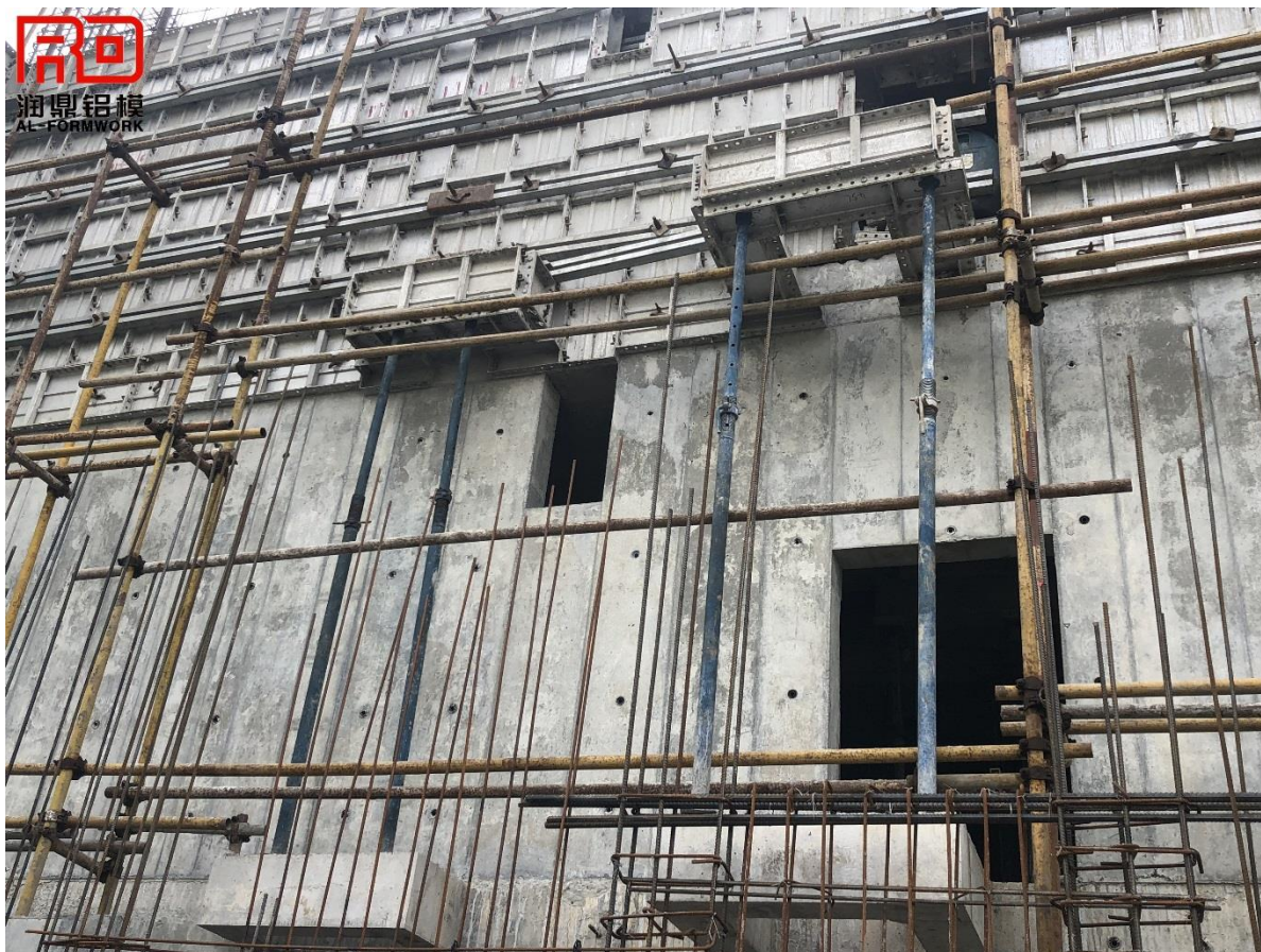
Protruding structure of external wall, aluminum formwork project.
