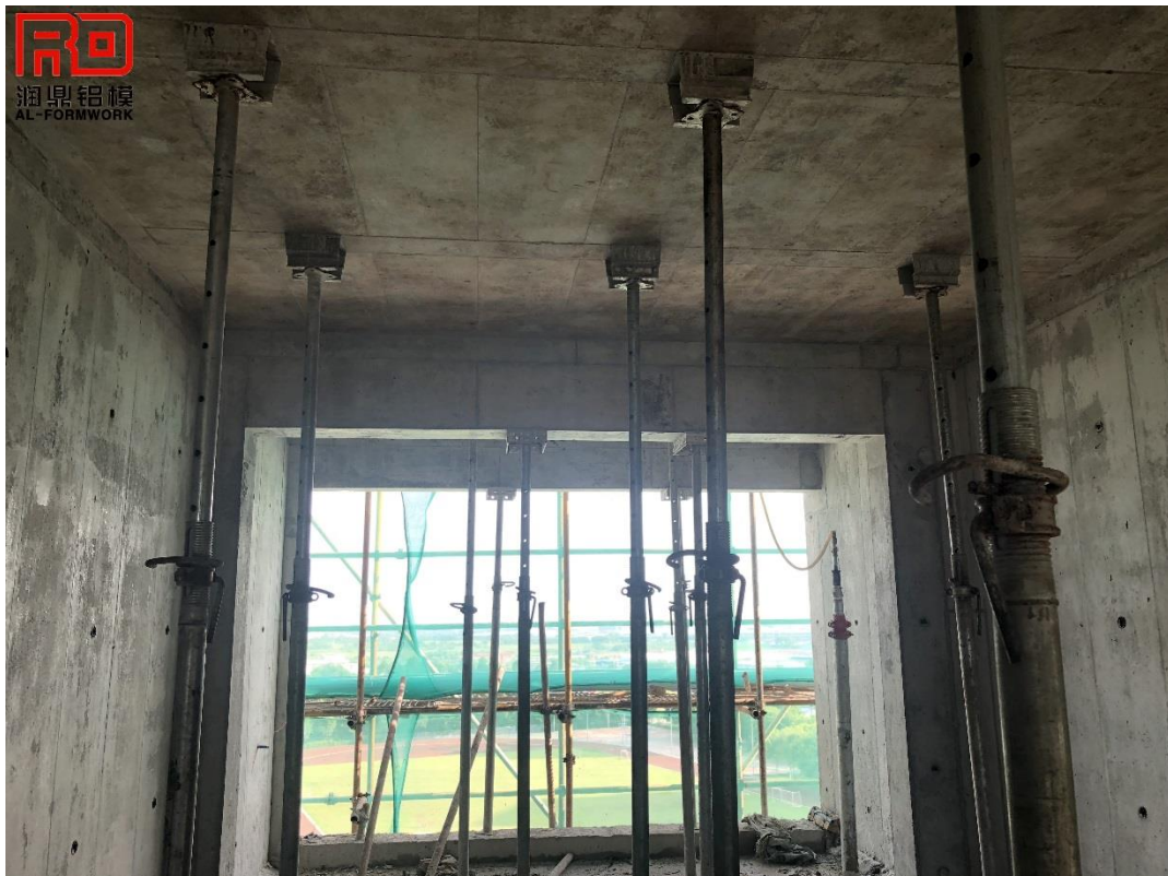
After 24~48 hours could remove all of alu-formwork panels, stayed supports only.
