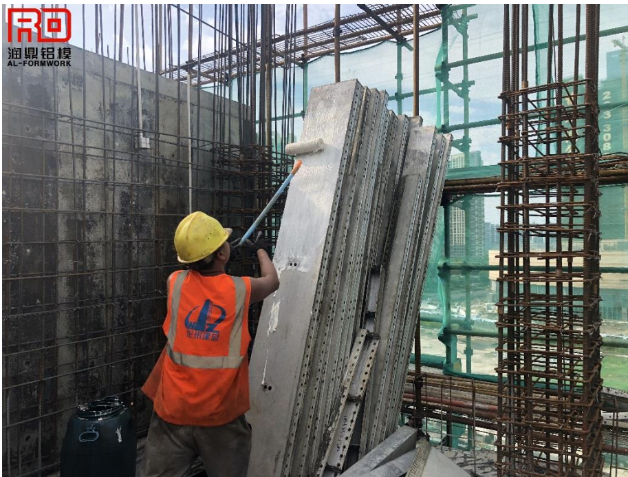
Coating the demoulding agent.
