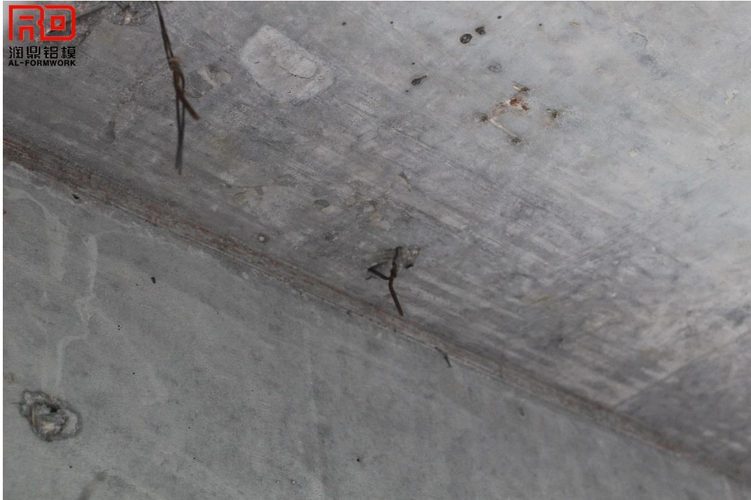
Iron nails stayed on the concrete surface.
