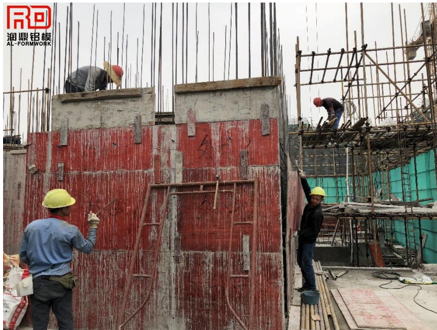
Plywood are fixed by iron nails with little wooden sheets
