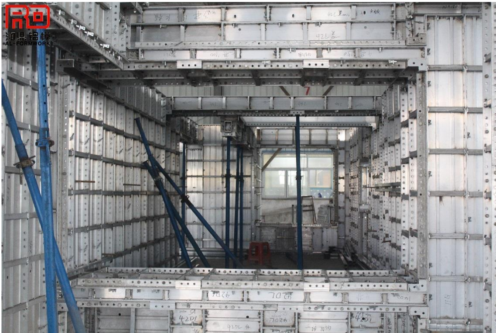
Pre-assemble the a whole set of alu-formwork system
