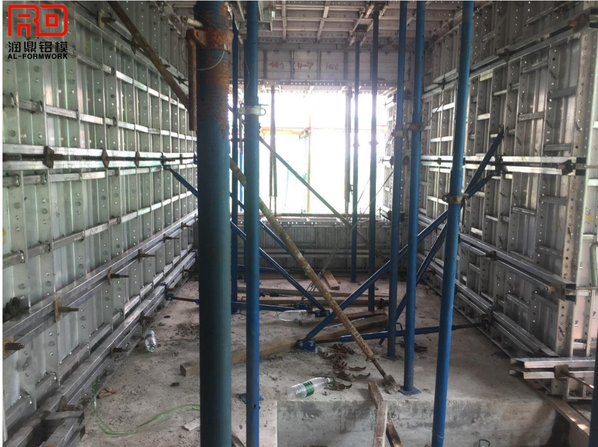
Aluminum formwork system could be set up all of structures
